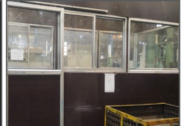
Dedicated Production office for shop floor Supervisors
